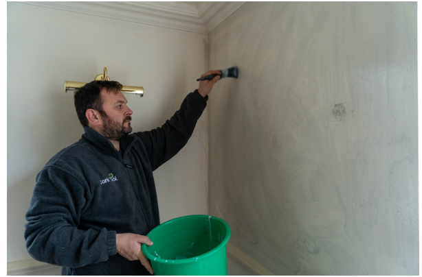
Application of quick drying primer
