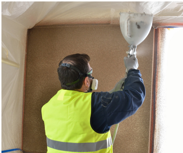
SprayCork application to walls in two coats
