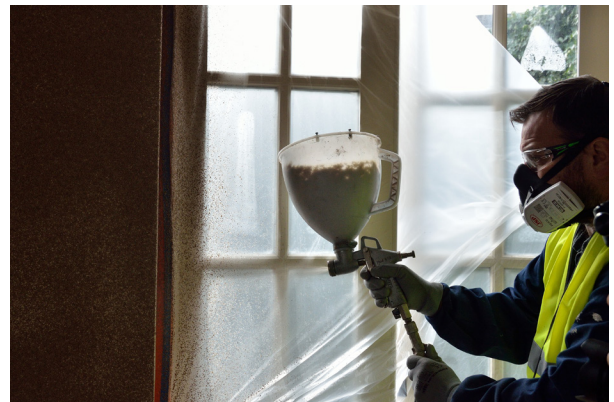
Continuous, seamless application around corners and window reveals
