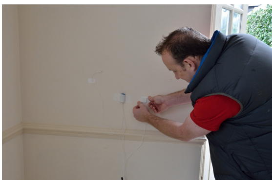
Interior set-up of U-value testing sensors before treatment
