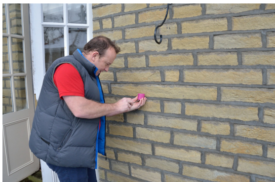
Exterior set-up of U-value testing sensors
