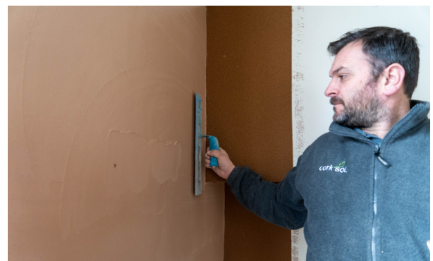
Plaster skim directly over the SprayCork
