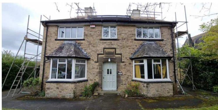
Figure 2. Front elevation of the property in the case study.
